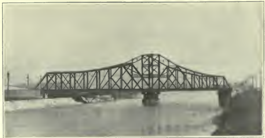
FIG. 266. BRIDGES. Swing bridge of the Illinois Central Railroad across the Sanitary Canal at Kedzie Avenue.
